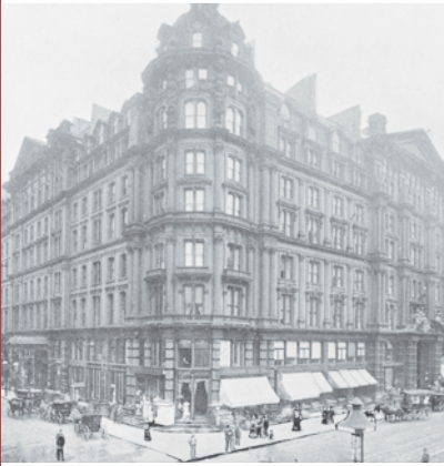
PALMER HOUSE, 1894 Chicago Public Library, Special Collections
